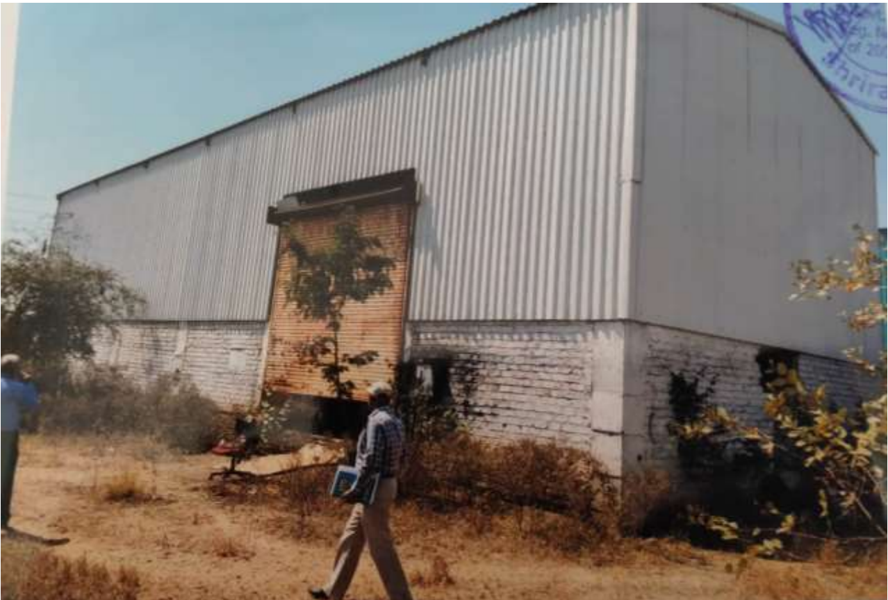
M/s. Ghuge Aditya Solar Industries Pvt. Ltd. - PLANT
