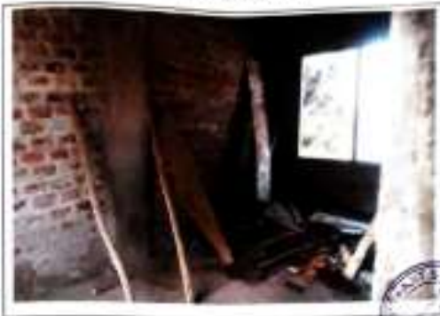
BEDROOM 1 ON FIRST FLOOR
