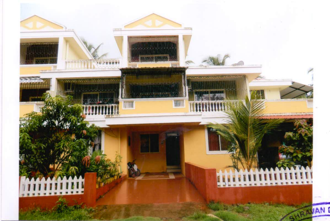
VIEW OF ROW HOUSE RH-2 FROM OUTSIDE
