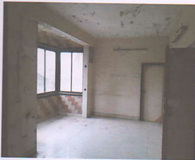
Photo Showing Living Area View
