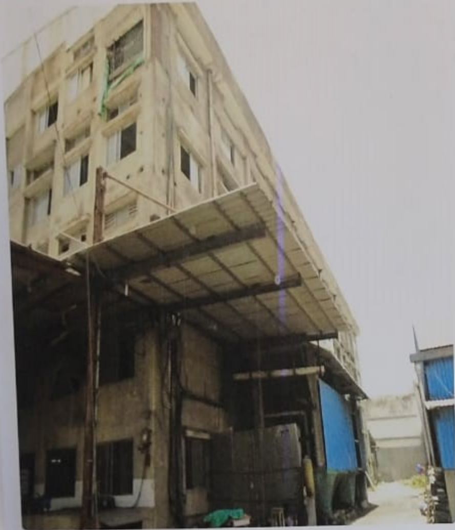
External view of the building
