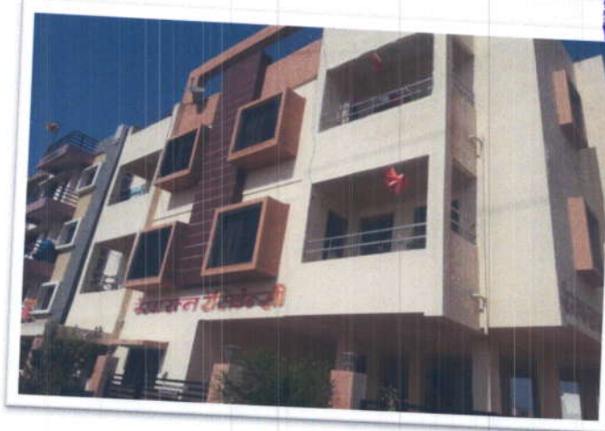
RESIDENTIAL FLAT NO. 104, SECOND FLOOR, "REKHARATNA RESIDENCY", OM NAGAR, GIRIRAJ VIHAR, SHEGAON – RAHATGAON ROAD, AMRAVATI, TQ, / DIST. - AMRAVATI, OF MR. VIJAY MADHUKAR CHOWDHARI.
